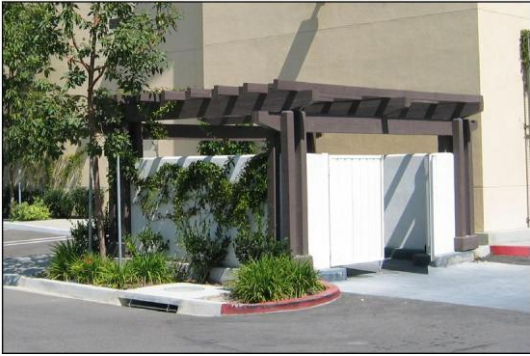
3.2.1.9 d) Screening of refuse containers and utilities is an inexpensive way to maintain the attractiveness of shared open space.
