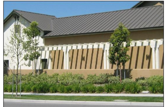
3.2.1.8 b) Low rise, landscaped screening walls contribute to a more attractive environment.
