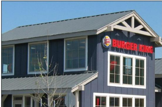
3.3.3.3 a) Exposed rafter ends, overhanging eaves, multiple roof planes and varied fenestration create interesting commercial buildings.
